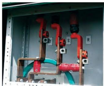
*Insulated rotary clamps provide a compact connection to a slotted busbar.*
